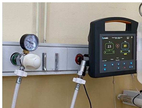
Figure 2. Installed O 2 matic.
